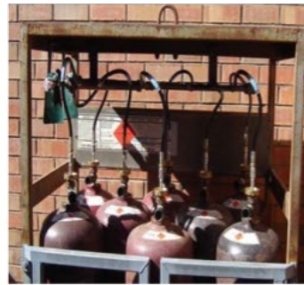
(a) Examples of manifolding of cylinders
