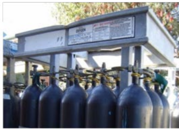
(a) Examples of manifolding of cylinders
